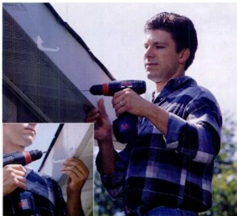
Mounting brackets for the Rainhandler Rain Dispersal System are attached to the siding fascia board below the roof's drip edge, then the louver sections simply snap into place.
