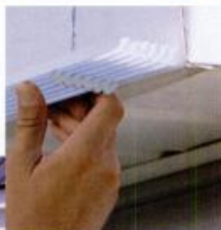
Mounting brackets for the Rainhandler Rain Dispersal System are attached to the siding fascia board below the roof's drip edge, then the louver sections simply snap into place.
